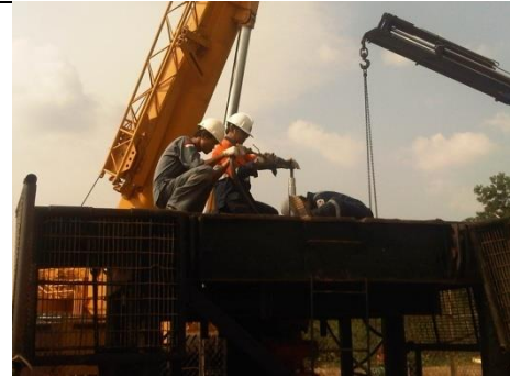
Figure 9 Execution of Drilling the Stuck Disk
