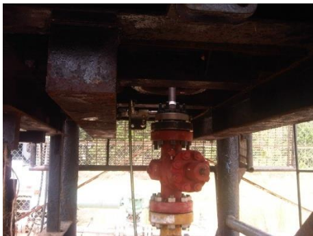
Figure 7 Installing Drilling Machine on Top of the Isolation Valve
