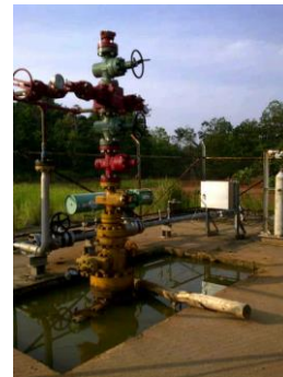
Figure 10 Well M-03 was Back on Production after Drilling the Stuck Valve
