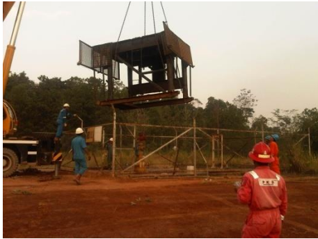
Figure 5 Setting Scaffolding (Rotary Table)
