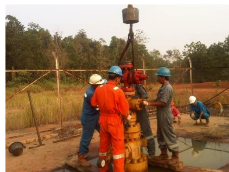
Figure 4 Installation of Isolation Valve on Top of the Stuck Valve
