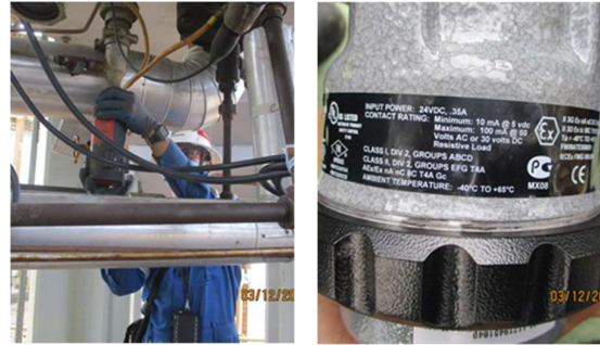
Figure 6 Execution Process at TOx
