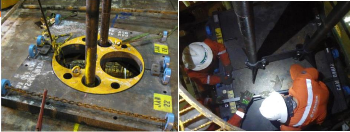
Figure 15 Make Up & Run in Hole Tubing Booster Line and Install CPPS
