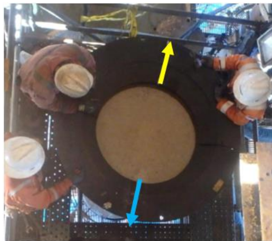
Figure 11 Install Funnel Entry Guide on Top CP
