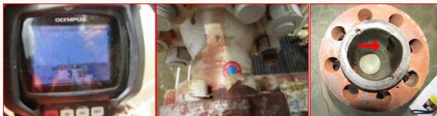
Figure 4 Sample case of severe choke erosion detected by iCIUT (minimum thickness at 30% from baseline)
