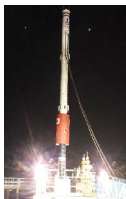
4. Pipe Hammering
