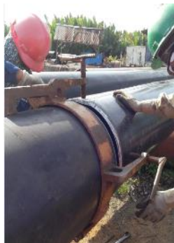
4. Pipe Hammering
