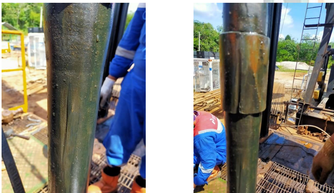
Figure 22 Tubing leak in Well GS-15
