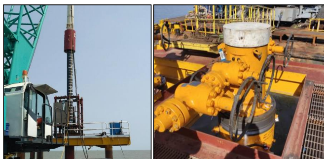
Figure 3. Rigless CP driving and actual CP & CWH after installation
