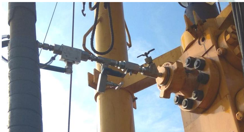
Figure 11. Connection of pumping line to ½” NPT in kill wing valve of TN-x
