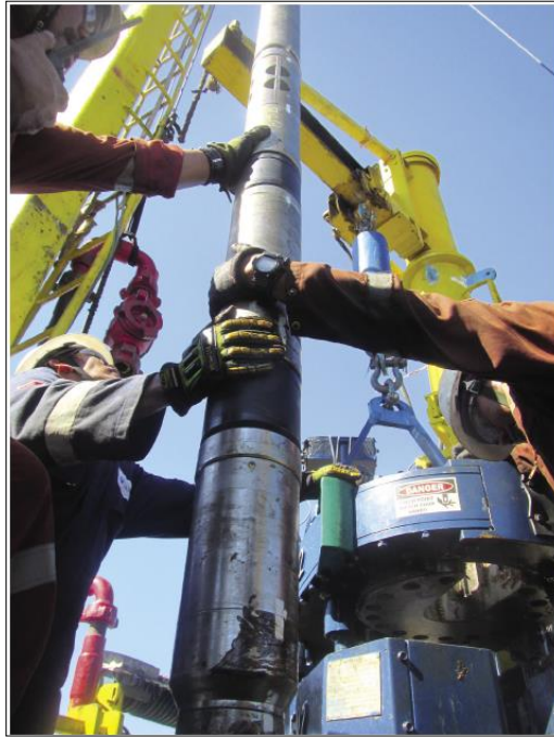
Figure 4 - Tubular Connection Process using Power Tong.
