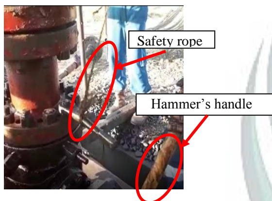
Figure 1 The Usage of Safety Rope as a Mitigation
